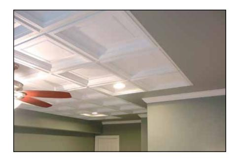
In perimeter and border situations where the T-bar sections are irregular or not a full 2' x 2' or 2' x 4' in size, edge trim styles can be easily trimmed to fit using common, household scissors.
